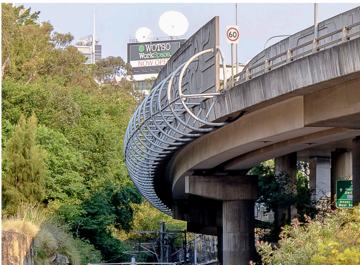
Reference Image - Galvanised steel support structure to precast concrete panels on the expressway.
